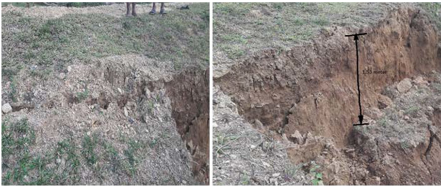
Fig. 11 Surficial slope failure at one of the ponds in Kumarghat, Tripura
