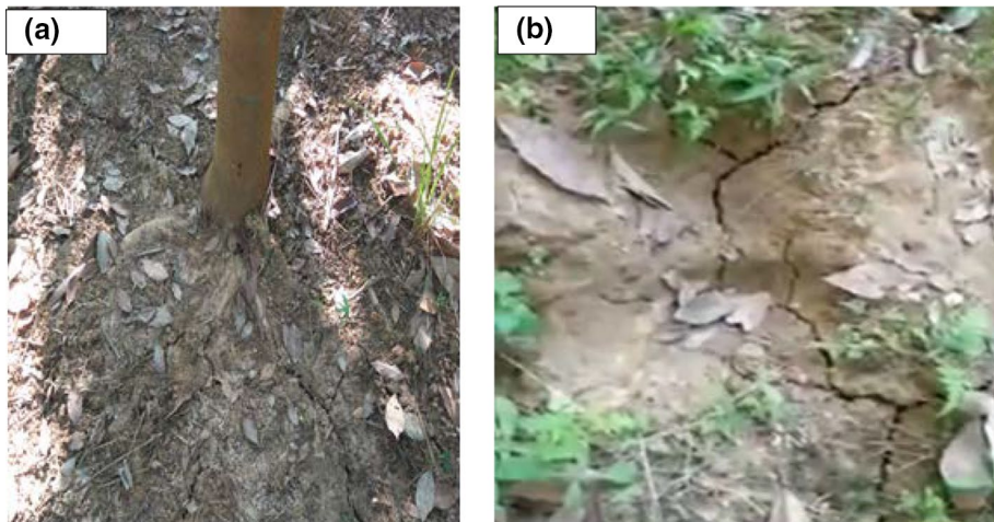
Fig. 21 a, b Surface cracks at the epicentral area located at the top hill of Longtharai, Dhalai, Tripura
